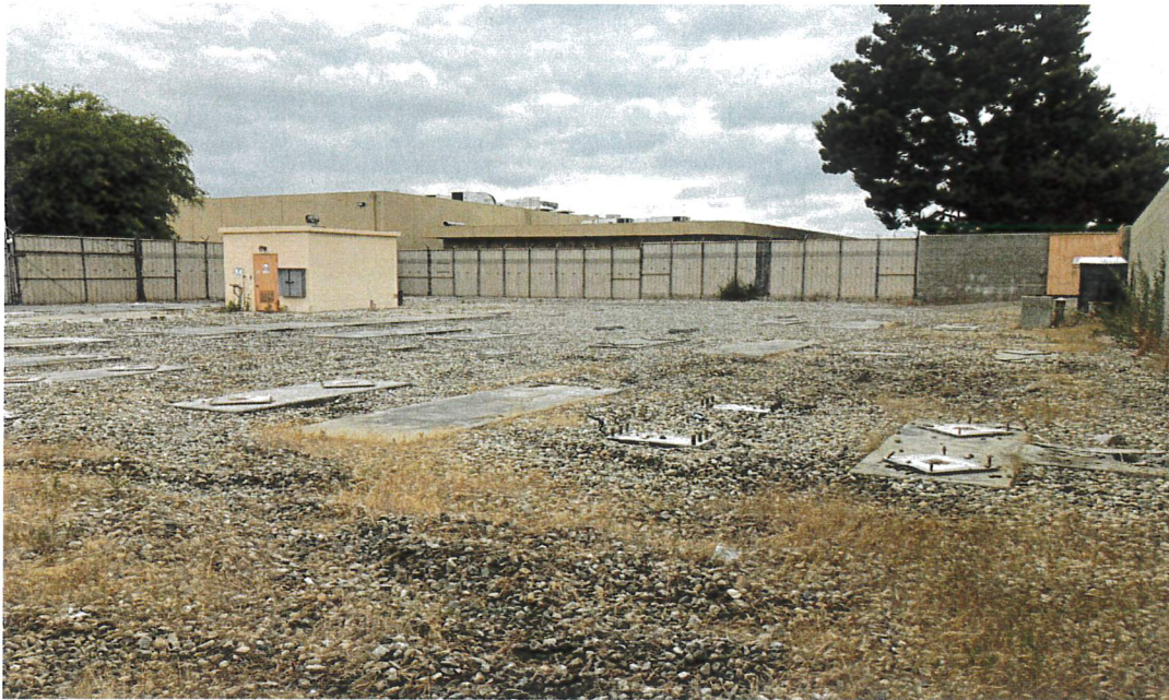
Pictures of the Pacific substation after the demolition
