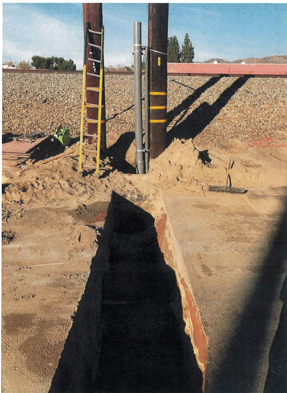
Installation of 69kV Riser Pole on Vanowen Street
