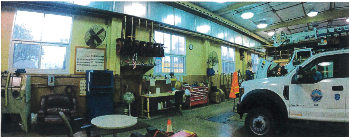
New, Insulated Windows with Operable Sections
