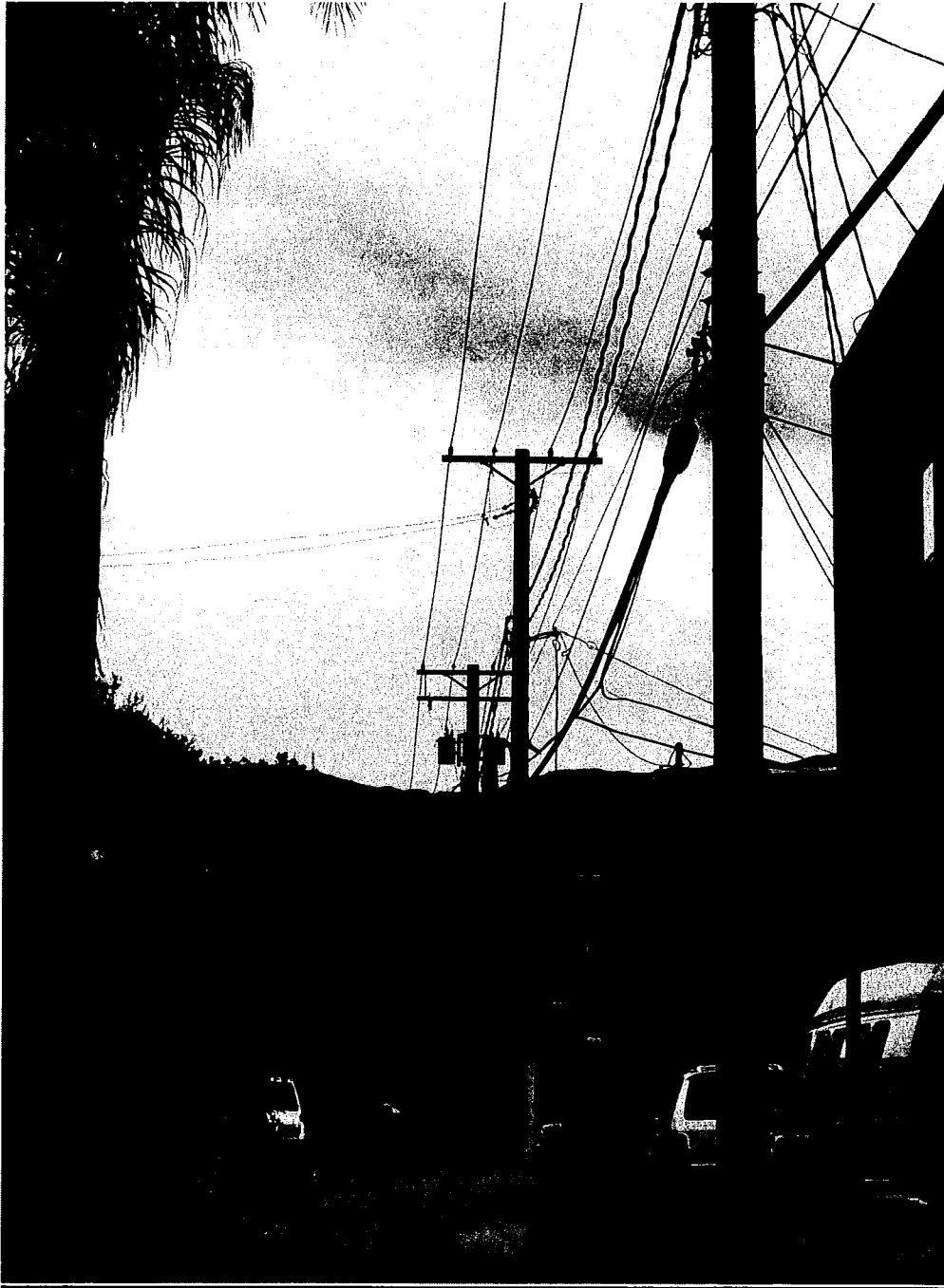
N-15 Alley Poles Set by Truck
