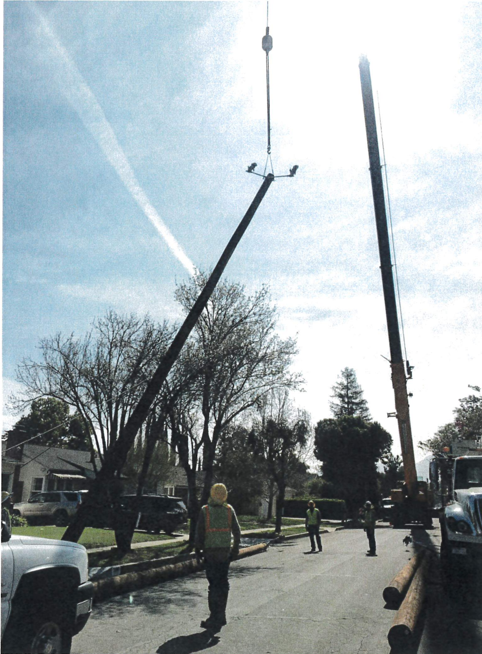
N-15 Property Line – Crane Pole Sets
