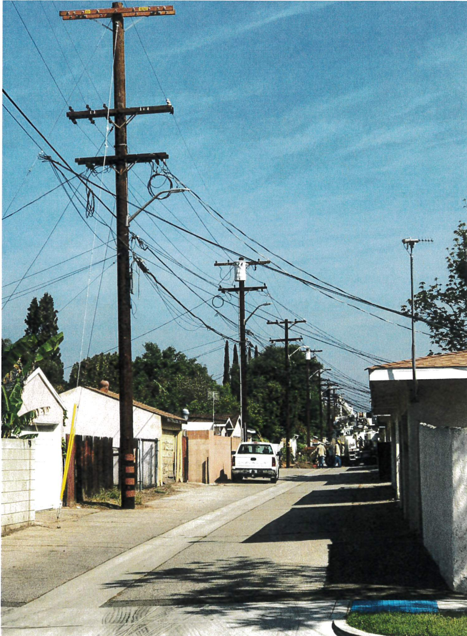
N-15 Alley Work
