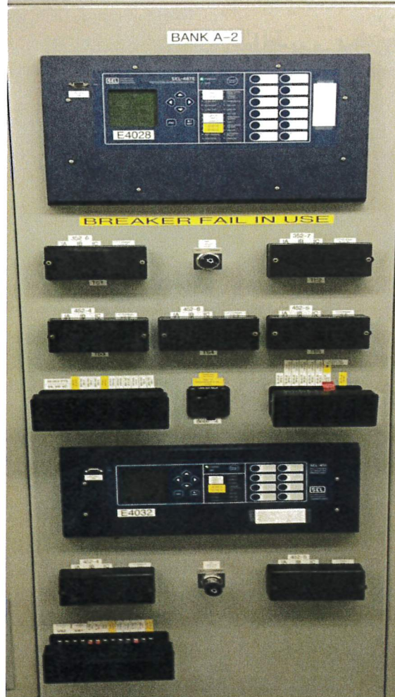
After Installation (New Relays)
