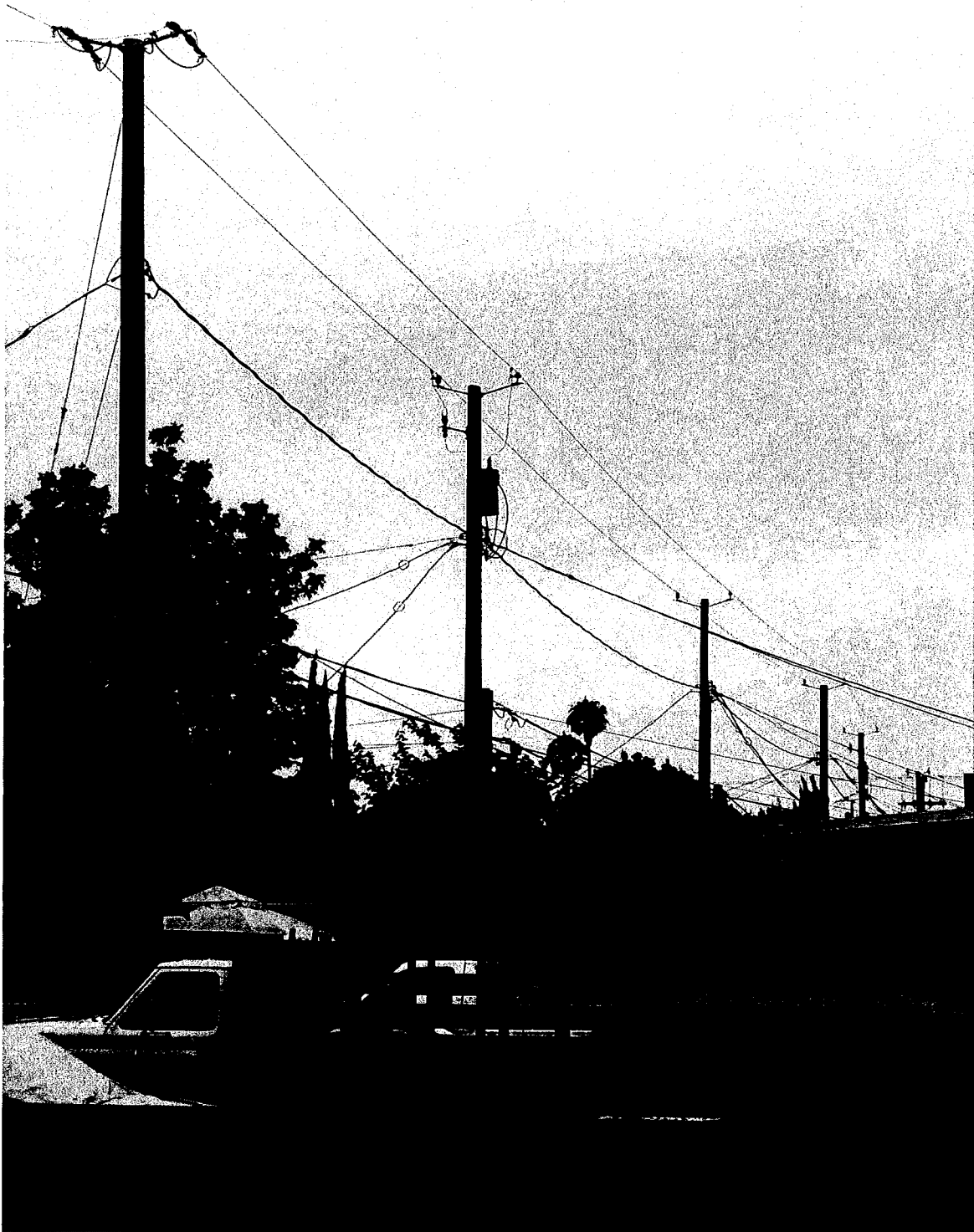
Property Line 12kV Rebuild
