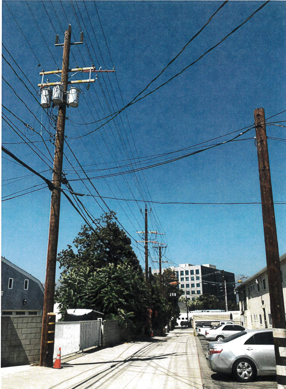
N-15 Alley Work
