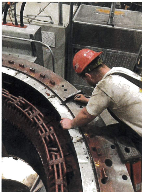
Unit 2 Generator Stator Inspection
