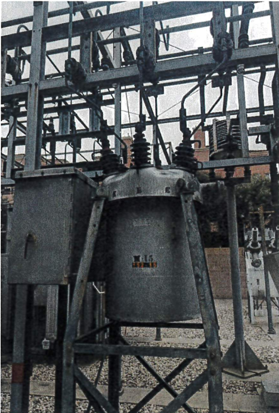
Original 4 kV Oil Circuit Breaker for McCambridge M-15
