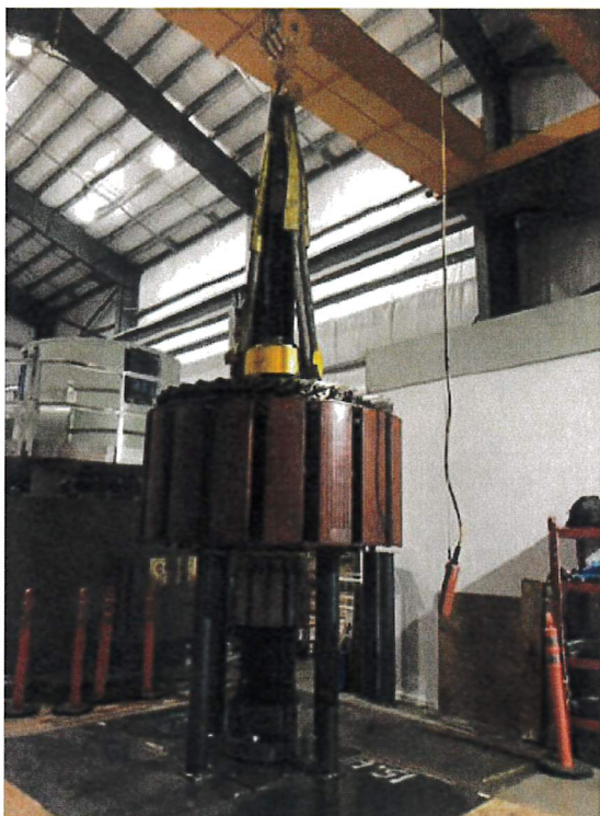
Unit 2 Generator Rotor Inspection
