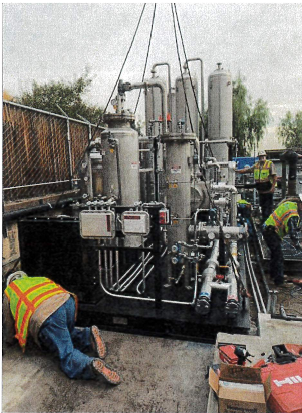
LFG Conditioning Skid
