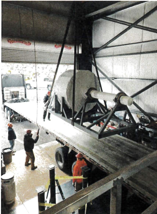
Unit 2 Generator Rotor Transport
