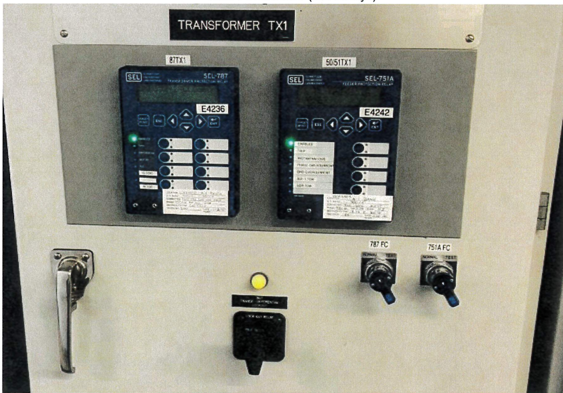
After Installation (New Relays)
