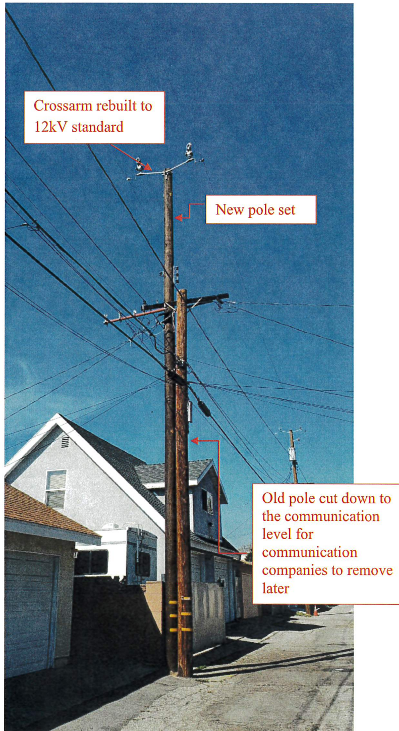
Progress of V-7 construction along alley east of N. Lincoln Street
