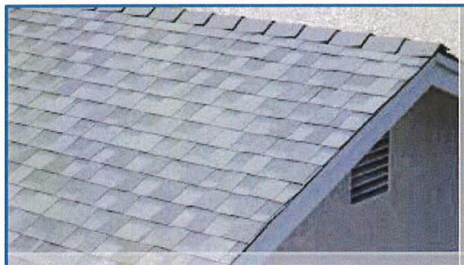
Figure 3. Composition Asphalt Shingle Roof
