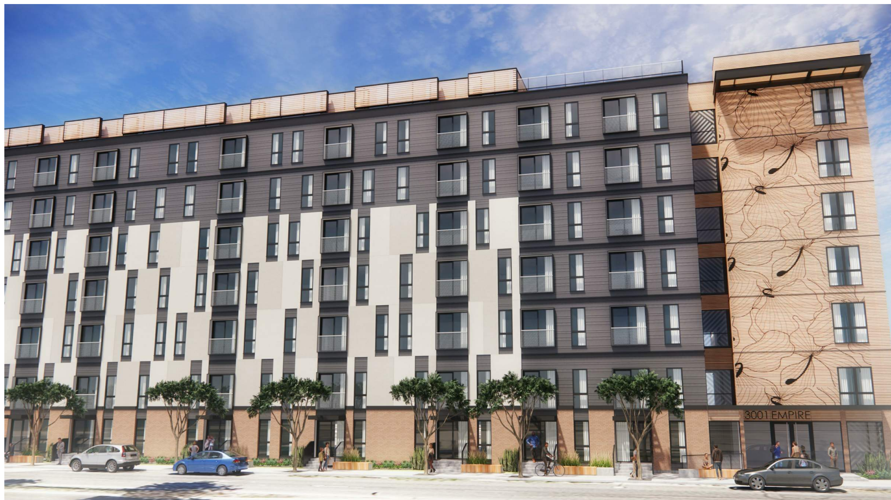
VIEW OF EMPIRE AVENUE FACADE
