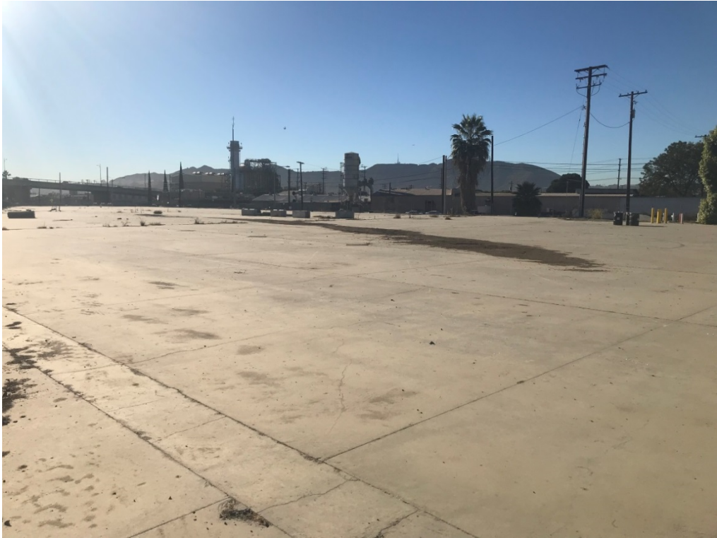
View of the vacant lot and former building pads
