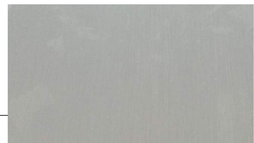
TILT-UP CONCRETE PANEL, PAINTED WHITE
