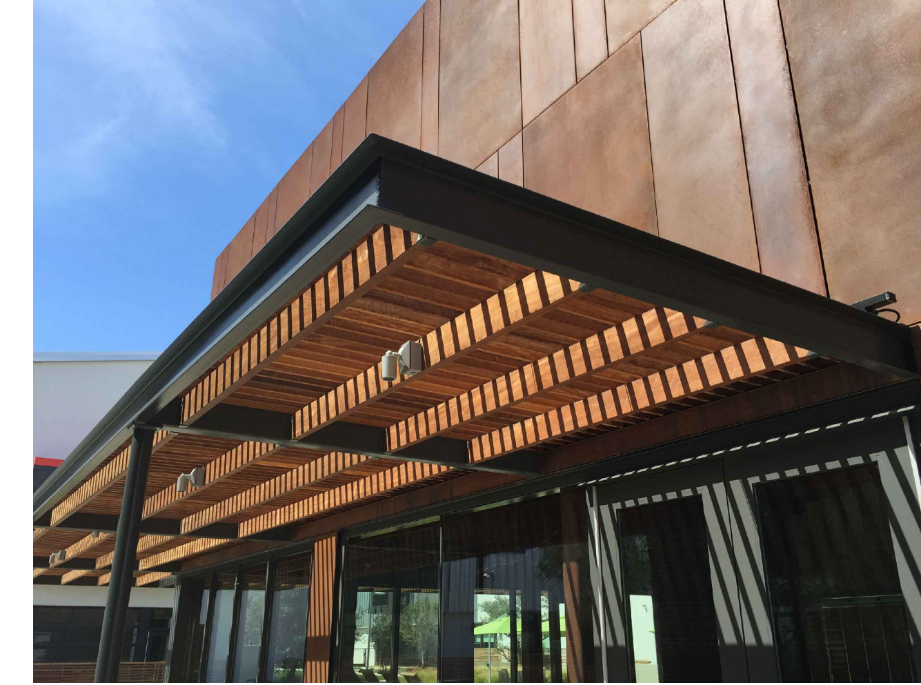
STEEL BEAM CANOPY WITH WOOD INFILL
