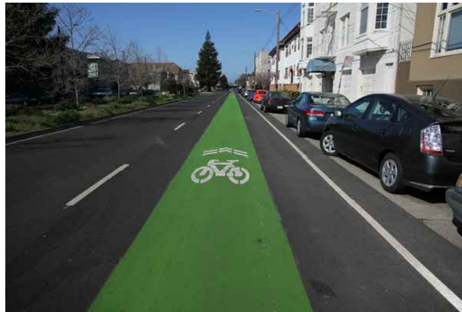
PAINTED BIKE LANE ON ASPHALT
