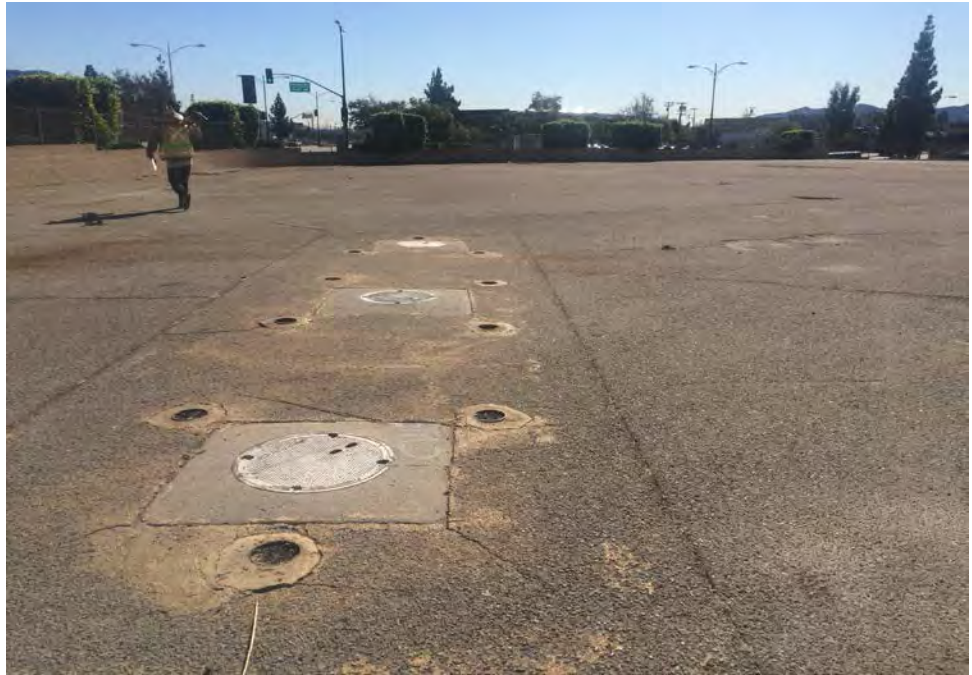
Photograph No. 5: View of groundwater monitoring well B-6-CW06 observed on the northeastern side of the property.
