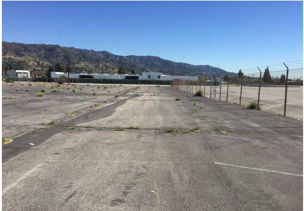
Photograph No. 3: Site, looking east.
