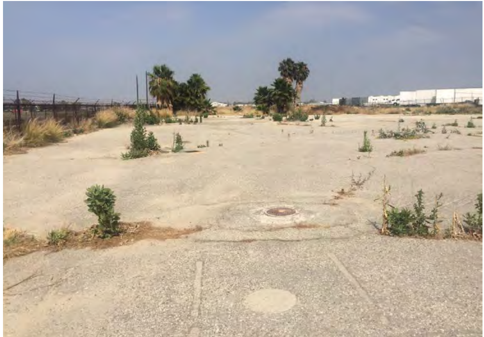
Photograph No. 3: View of the site, looking west from the entrance. Monitoring well MW-1 in foreground.
