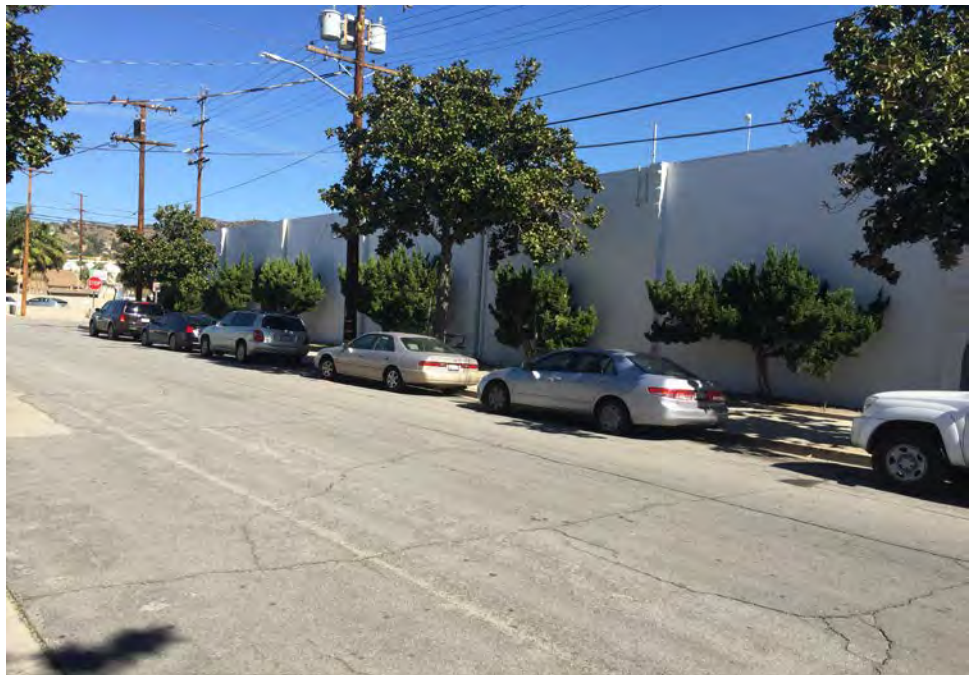
Photograph No. 6: Commercial building located immediately north of the site.
