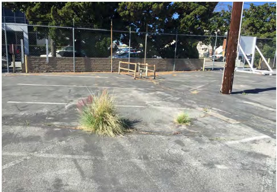
Photograph No. 4: Vertical pipe used to hold a former canopy or sign, looking west.
