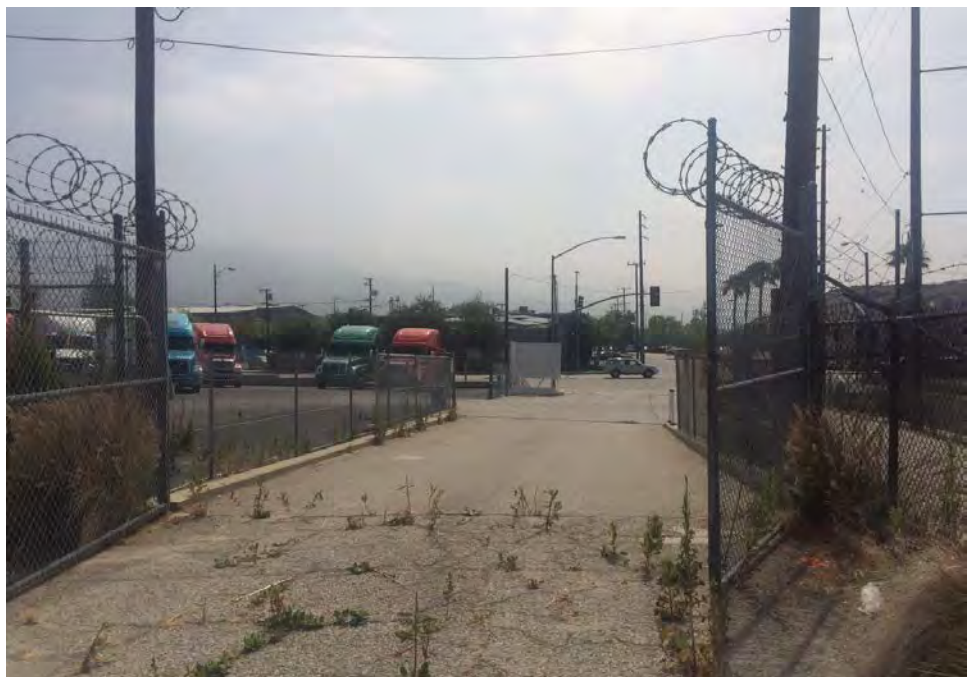
Photograph No. 2: View of the site entrance, looking east.
