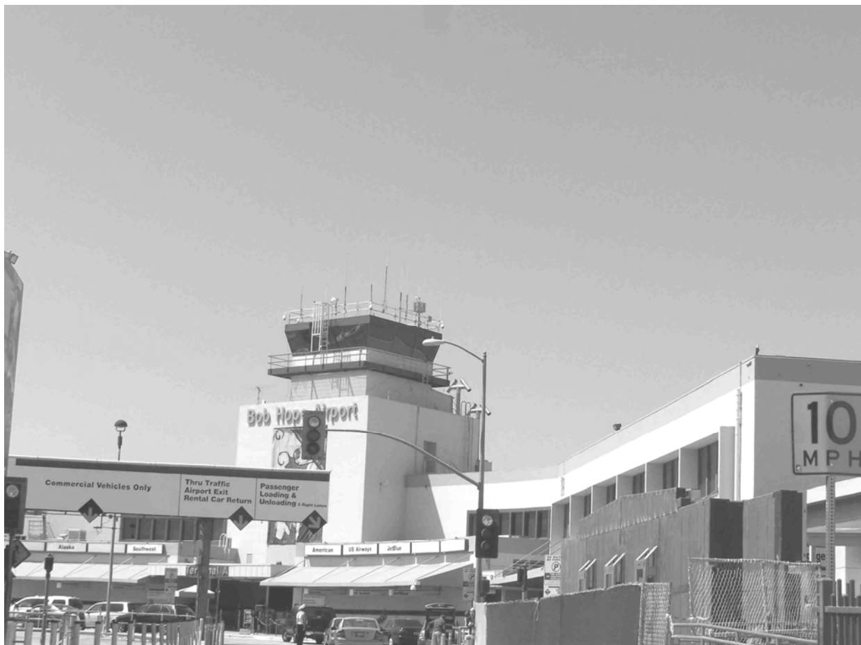
Figure 40. Current (2009) view of the (now) Bob Hope Airport terminal building that has been altered. (Photo taken by Galvin Preservation Associates, March 2009.)
