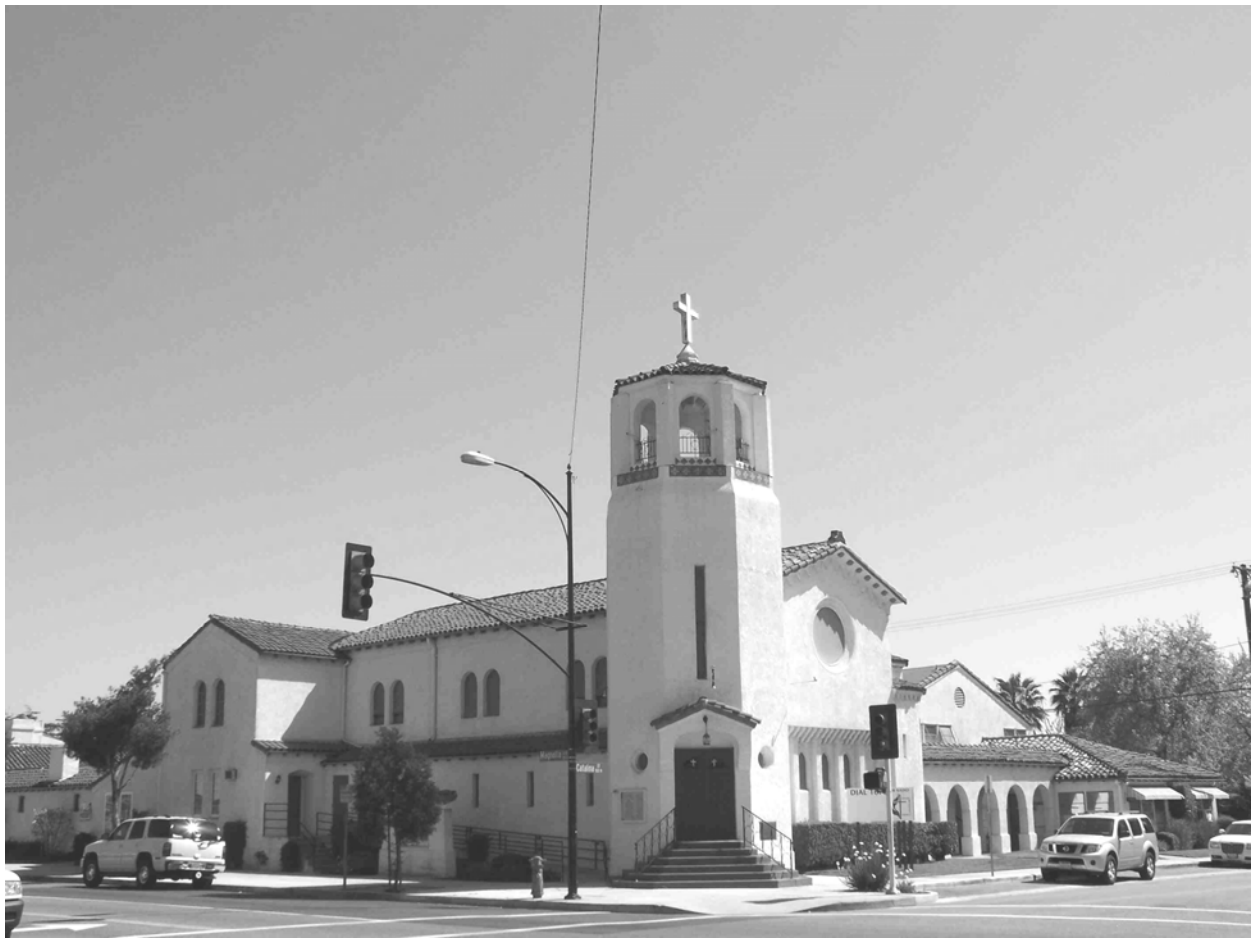
Figure 33. View of the Magnolia Park Methodist Church (Photo taken by Galvin Preservation Associates, March 2009.)
