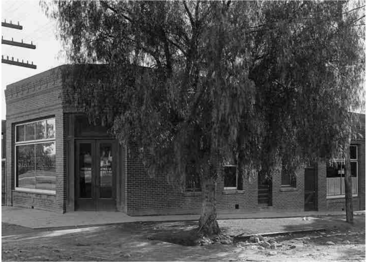
Figure 15. Circa 1908 view of the Burbank State Bank Building. (Los Angeles Public Library)
