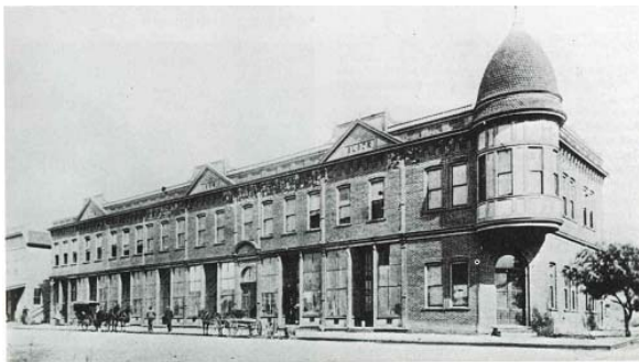
Figure 12. Brick clad downtown commercial building constructed in 1889 (E. Caswell Perry. Burbank, An Illustrated History , Northridge, CA: Windsor Publications, 1987).
