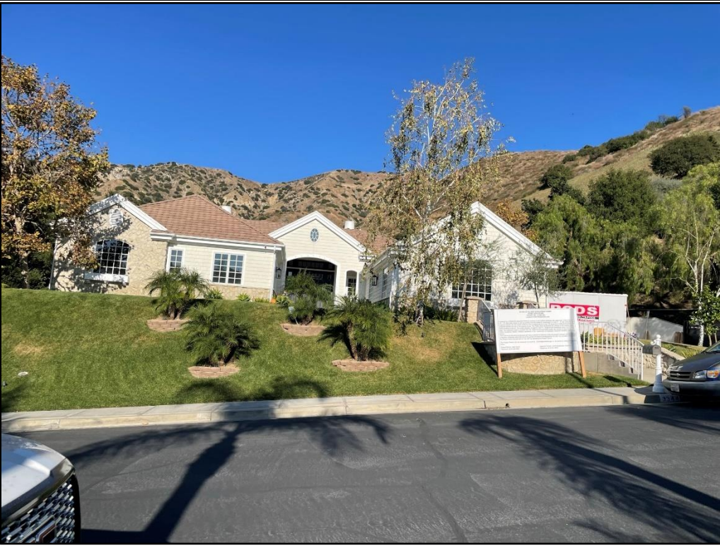
View from across Wedgewood Lane of the subject property.
